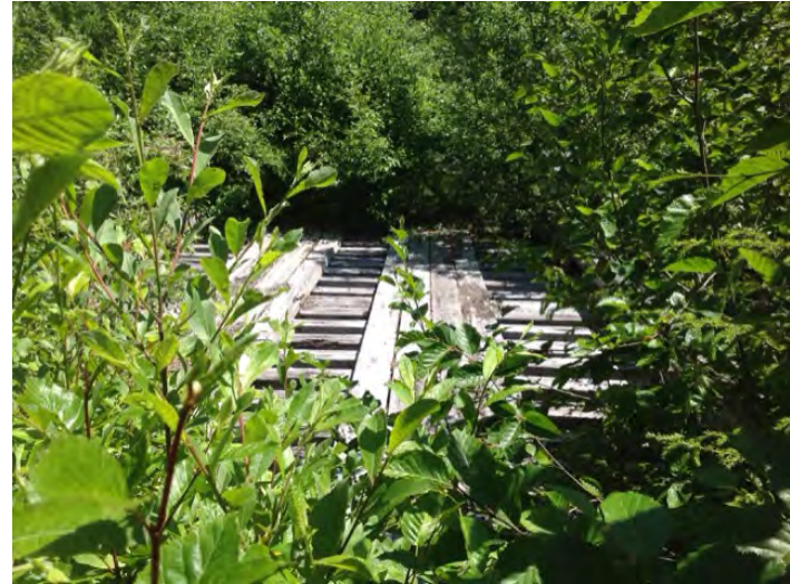
Approach from Left Bank when facing downstream
