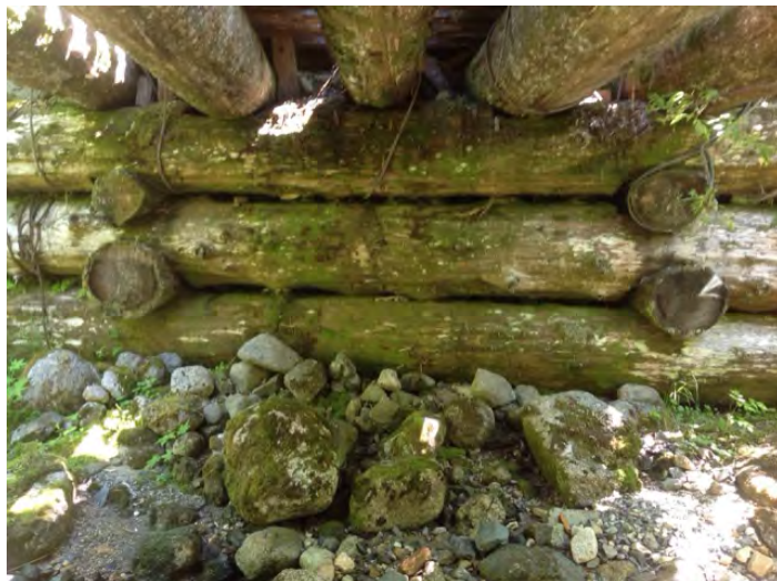
Right Bank Abutment when facing downstream
