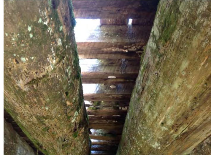
deck from below
